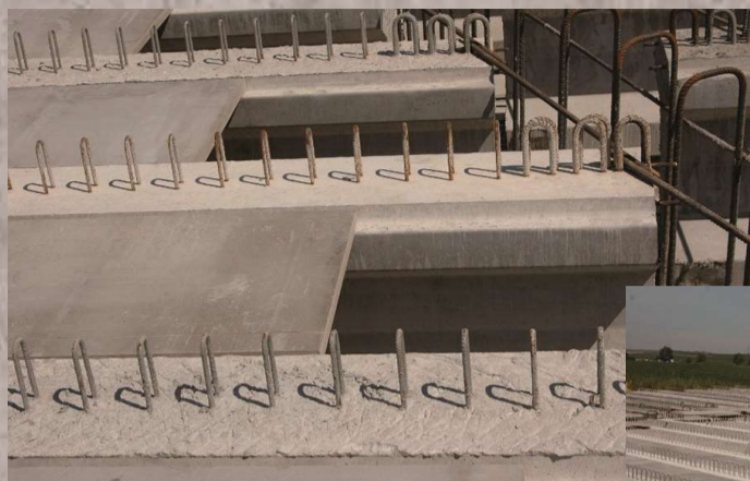
BETONYP ® as formwork
